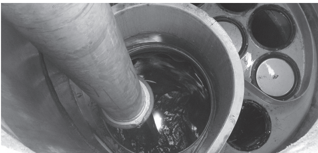
Vacuuming Sump Through MAW
